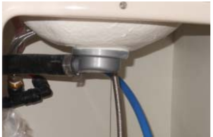
Head Sink Plumbing
